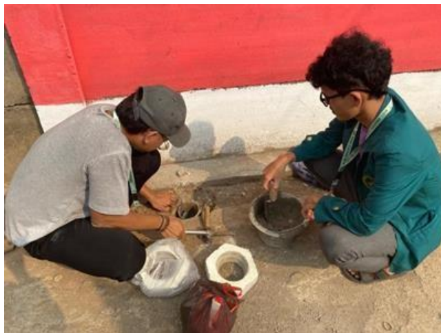
Figure 2. Installation of a 4-inch pipe into the biopore soil hole
