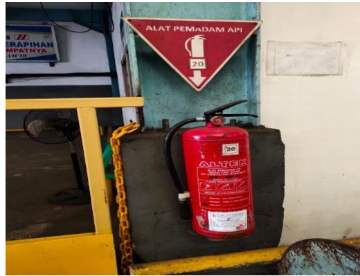
Figure 5. Installation of the fire extinguisher
