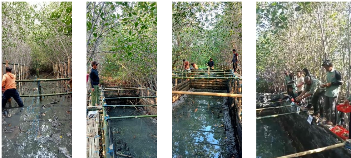
Figure 4. Silvofishery pond construction for mangrove crab cultivation
