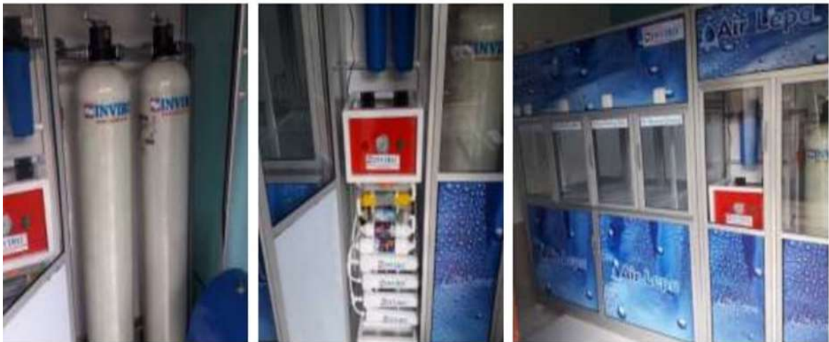
Figure 14. Reverse Osmis (RO) technology, which is used for drinking water treatment
