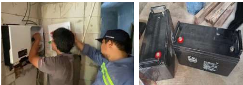
Figure 8. Hybrid Inverter and Battery Installation
