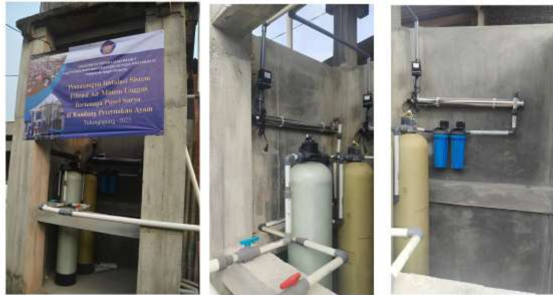
Figure 3. Placement of water filters below water reservoir buildings
