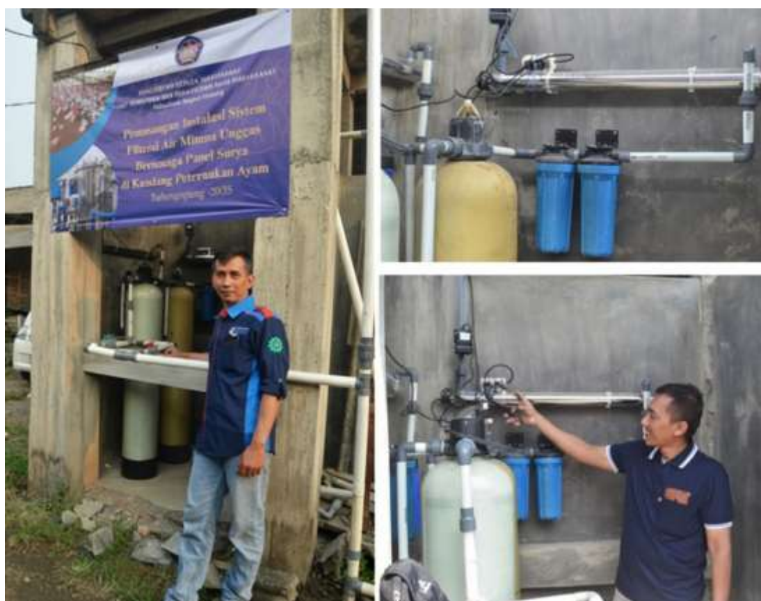
Figure 4. Filtration system for drinking water in poultry houses
