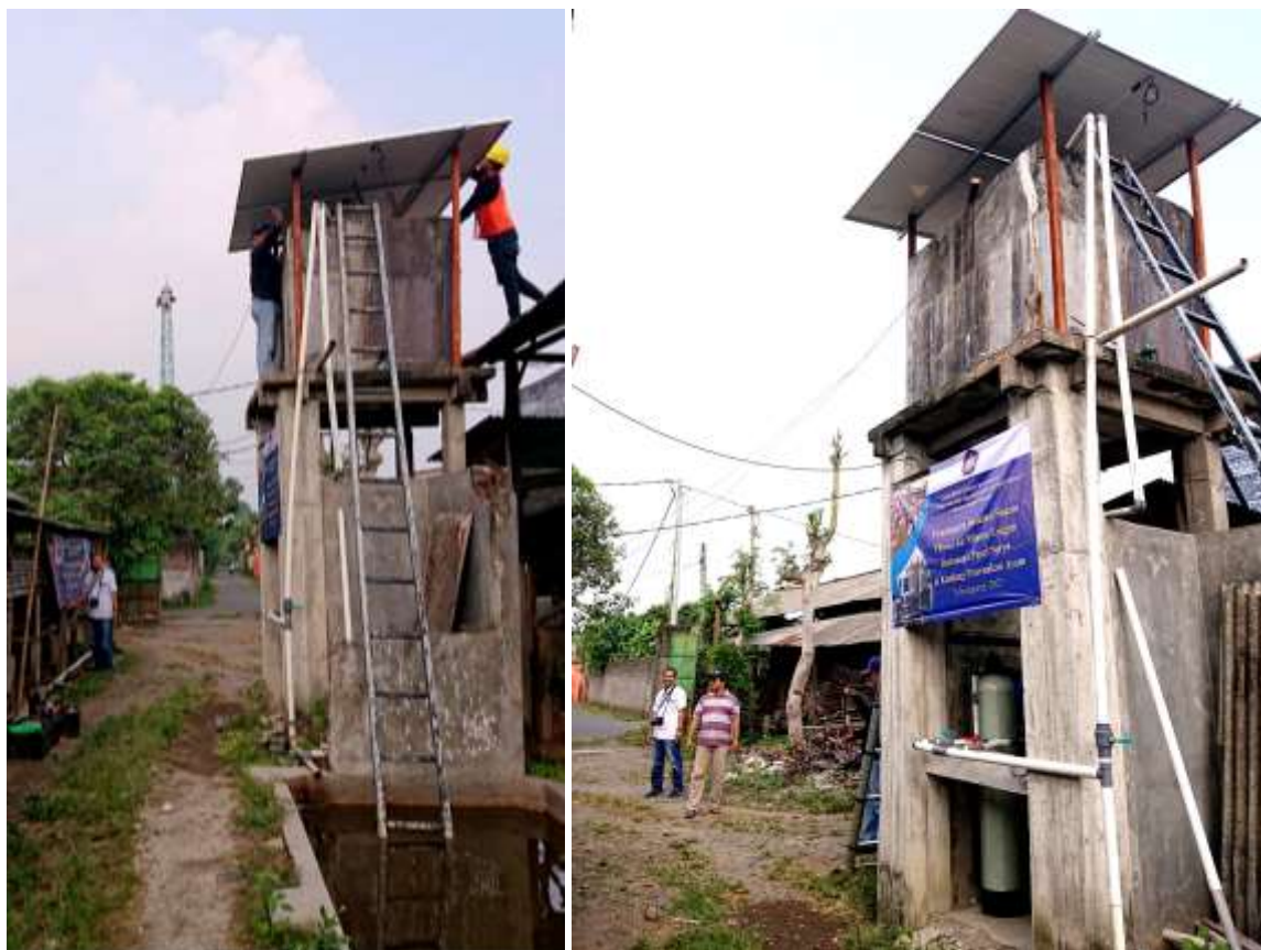
Figure 5. Positioning of solar panels above the water reservoir building
