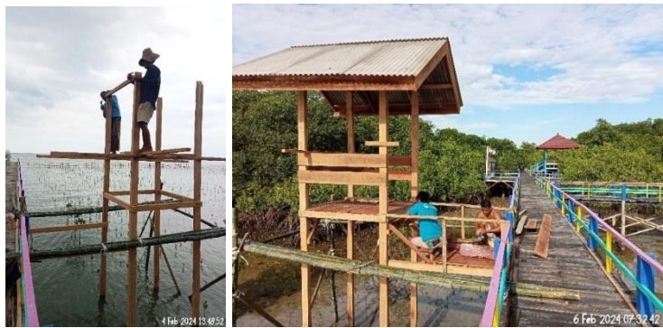
(c) Gazebo construction
