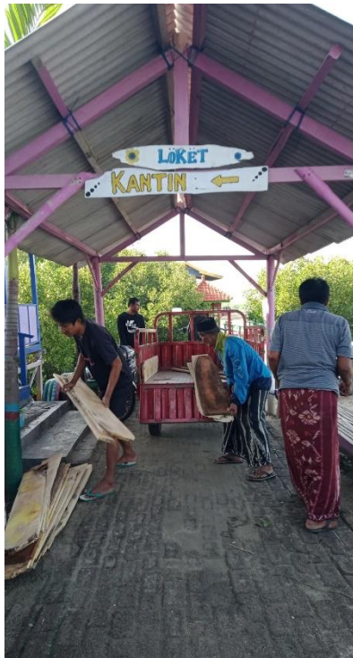
(b) Construction of tourist restaurants
