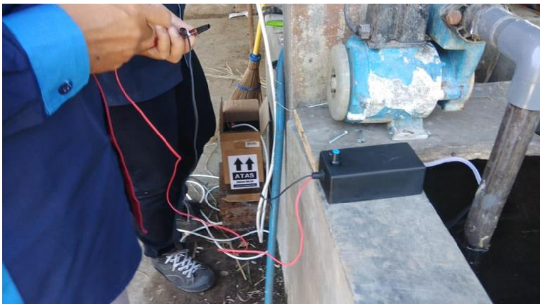
Figure 9. Pond aeration installation
