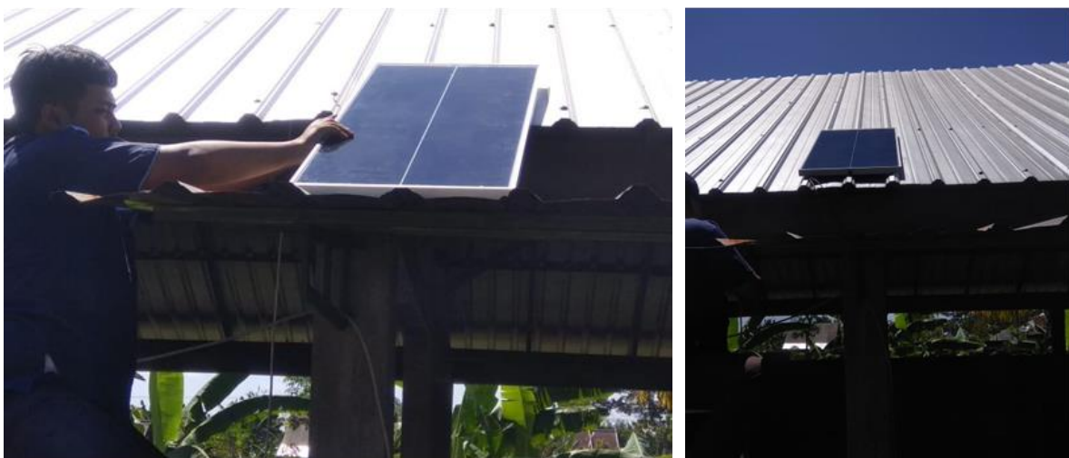
Figure 7. Mounting solar panels on a sloped roof
