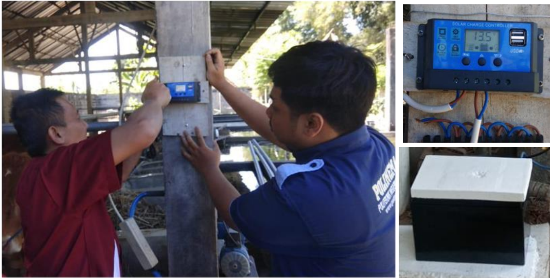
Figure 8. Installation of solar power equipment
