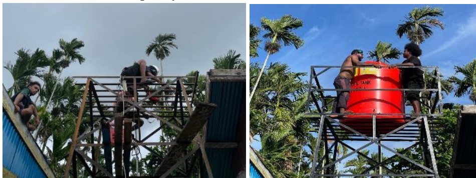
Figure 5. Assembly of the frame, pipes and tower supports
