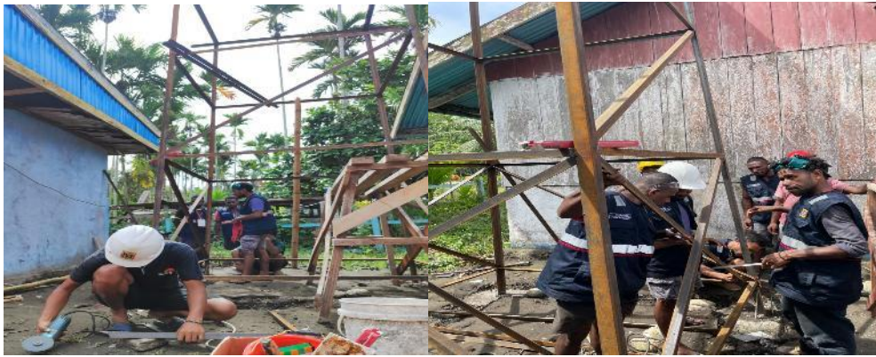
Figure 4. Construction of tower frame
