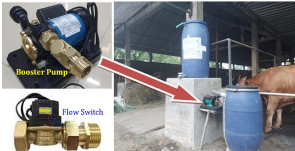
Figure 7. Installation and positioning of booster pump equipment
