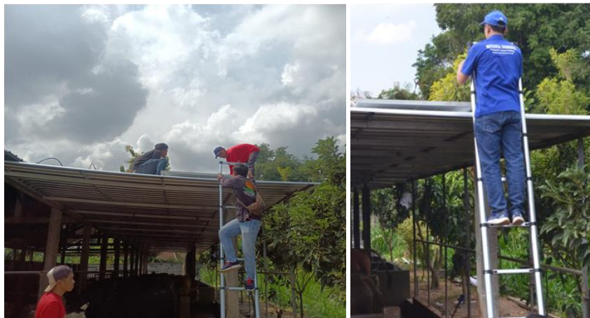
Figure 3. Installation of 540 Wp solar panels on the cattle shed roofs
