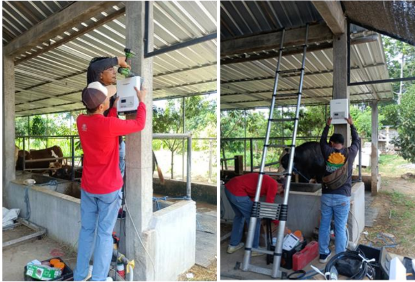
Figure 4. Installation of solar energy converters and their equipment
