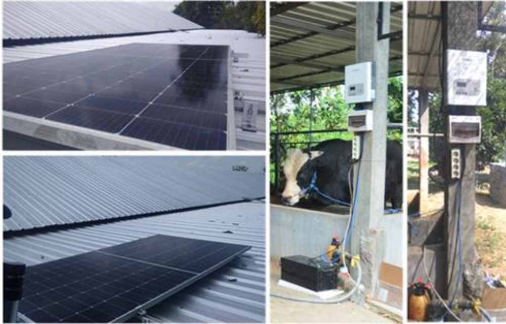
Figure 6. Results of the solar power system installation
