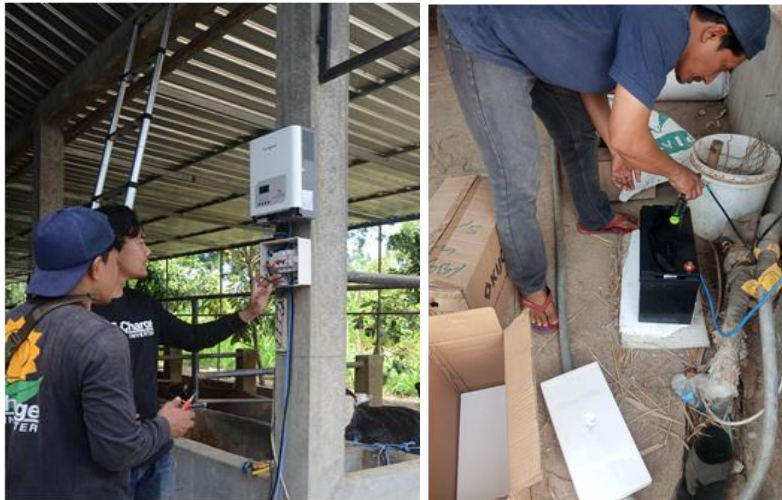
Figure 5. Installation of MCB panels & batteries
