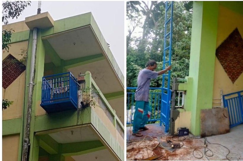
Figure 2. Construction of Maintenance Stairs at Solar Power Plant
