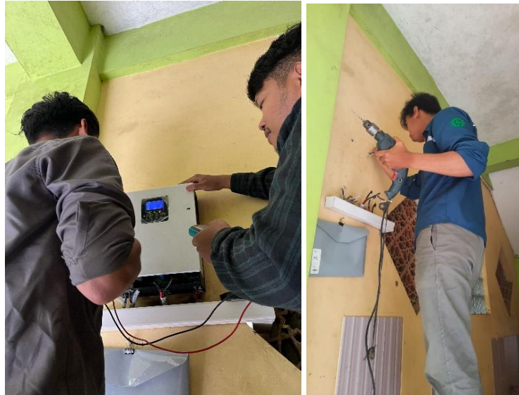
Figure 4. Installation of Inverter in Solar Power Plant
