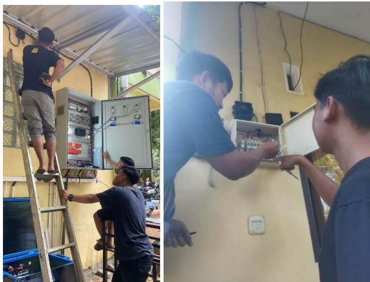
Figure 5. Installation of Load Panels on Solar Power Plant
