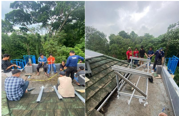
Figure 1. Design and Construction of Solar Power Plant Frames
