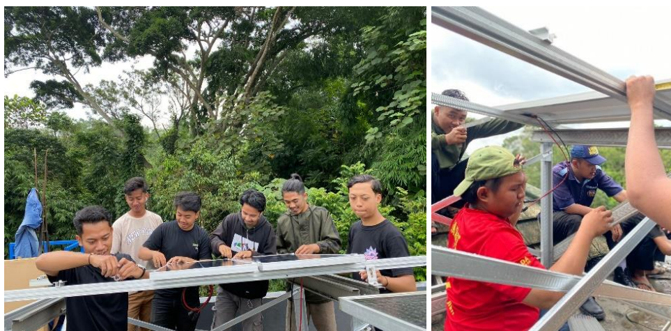
Figure 3. Installation of Solar Panels on Solar Power Plants
