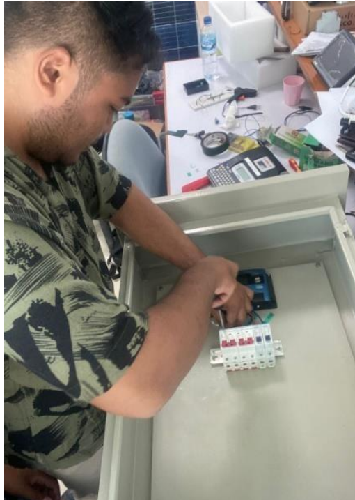
Figure 6. Panel Box Installation
