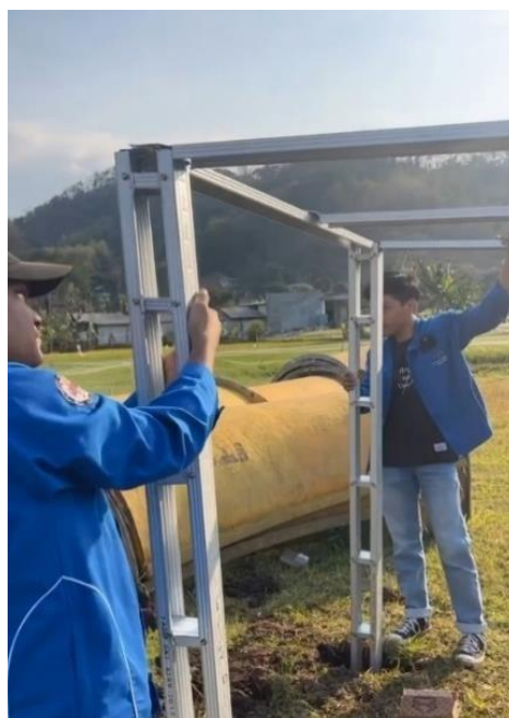
Figure 7. Installation of Mast Framed
