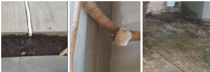
Figure 2. Air conditioning wastewater is wasted, causing moss and the roads to become slippery
