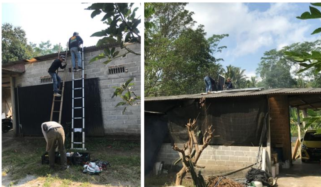
Fig.5 The installation of solar panel on the coop roof
