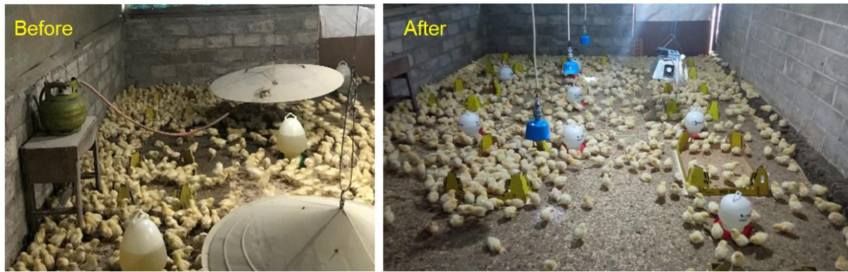
Fig.4 The DOC coop before and after the electric heater was installed
