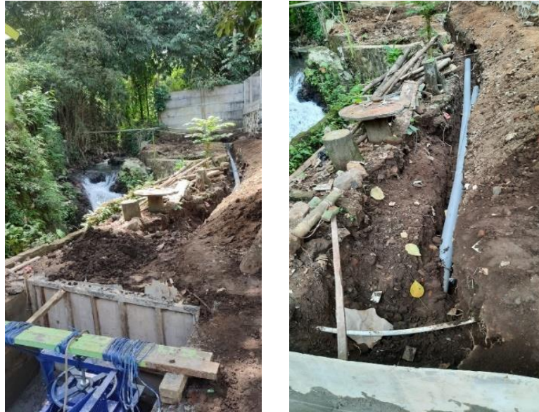
Figure 4. Installation of the PHPP Pipes
