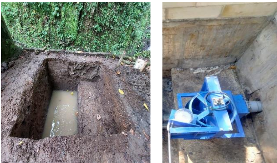
Figure 5. Construction of the PHPP Turbine Tank
