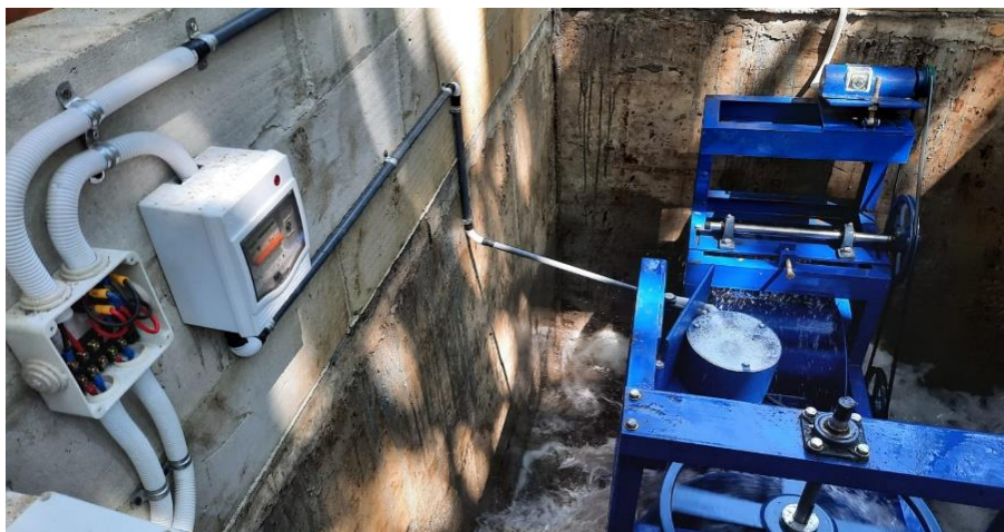
Figure 7. Installation of a 3 Phase AC Generator
