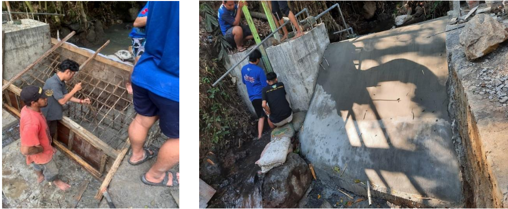
Figure 2. Construction of the PHPP Dam
