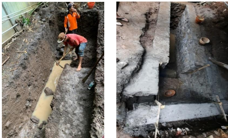
Figure 3. Construction of the PHPP Canal
