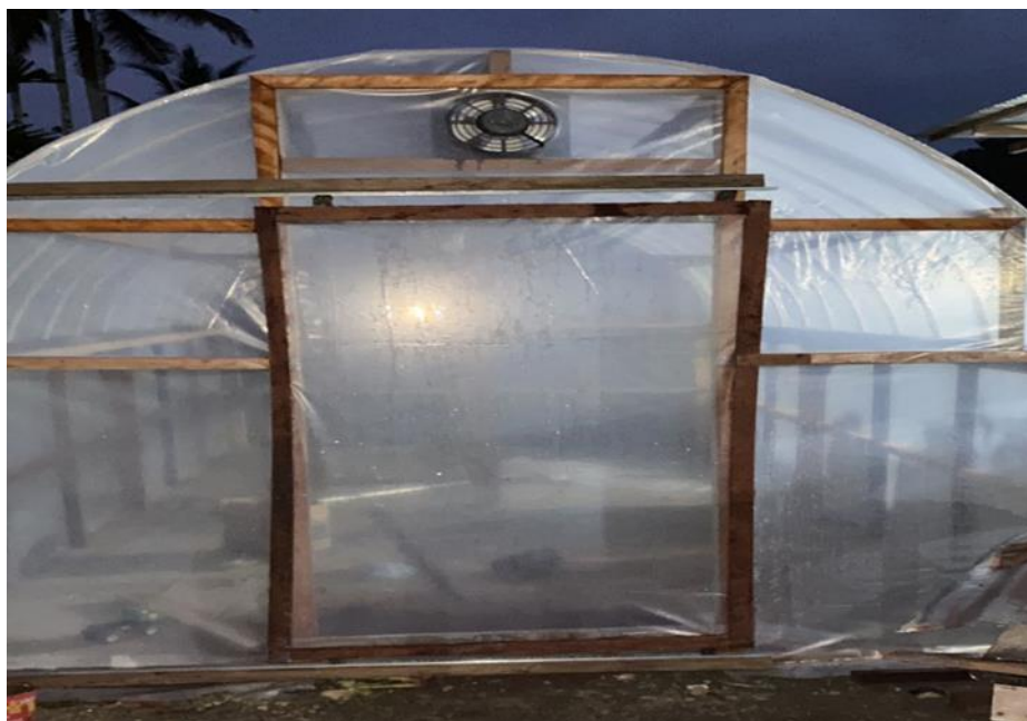
Figure 3. Complete construction of corn dryer
