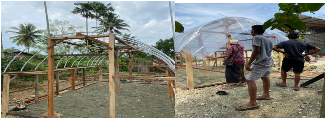
Figure 2. The activity of making a corn dryer
