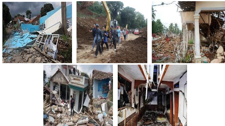
Figure 1. Damage to residents' houses and landslides in the village of Cugenang sub-district
