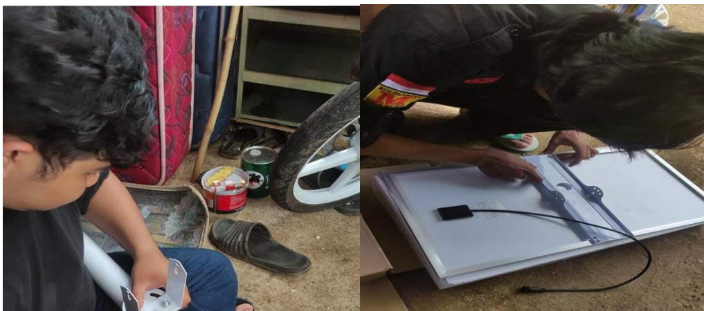
Figure 7. The process of installing solar cell light
