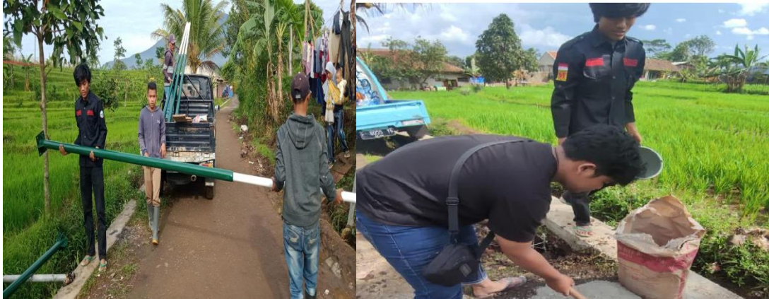
Figure 7. The process of mobilizing and installing solar cell PJU lights
