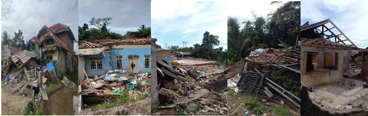
Figure 1. The current condition of the Cianjur Earthquake in the village of Nagrak, Cugenang District, Cianjur Regency
