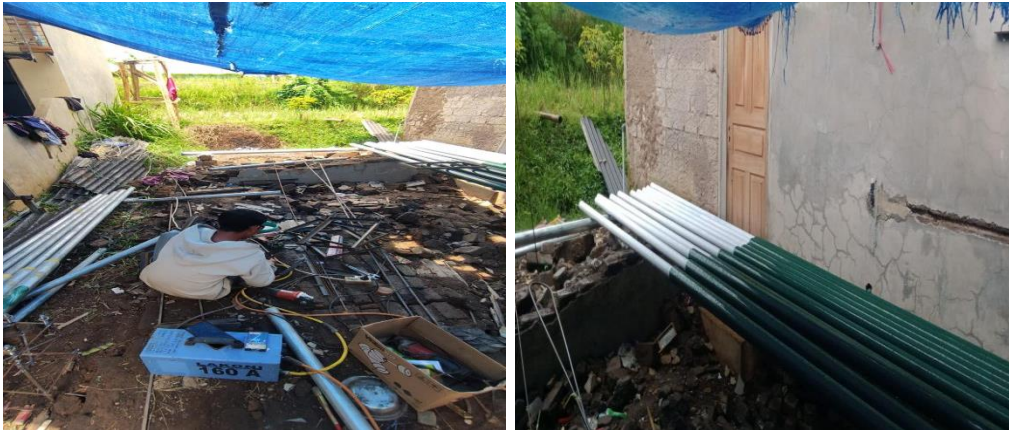
Figure 6. Pole manufacturing process
