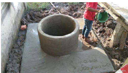
Figure 1. The Process of Making Dug Wells Source: Community Service Activity Report
