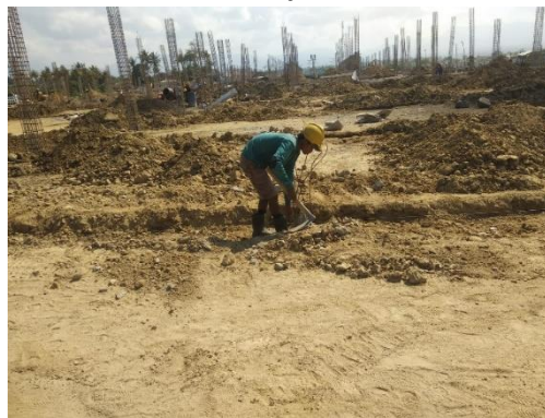
Figure 3. Workers Excavation for Sloof
