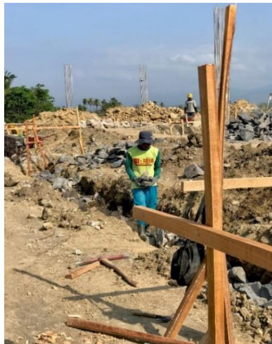
Figure 1. Workers working on river stone foundations Activity Location Sources
