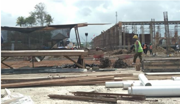
Figure 7. Workers at Work Carrying Out Sand Transport Activity Location Sources
