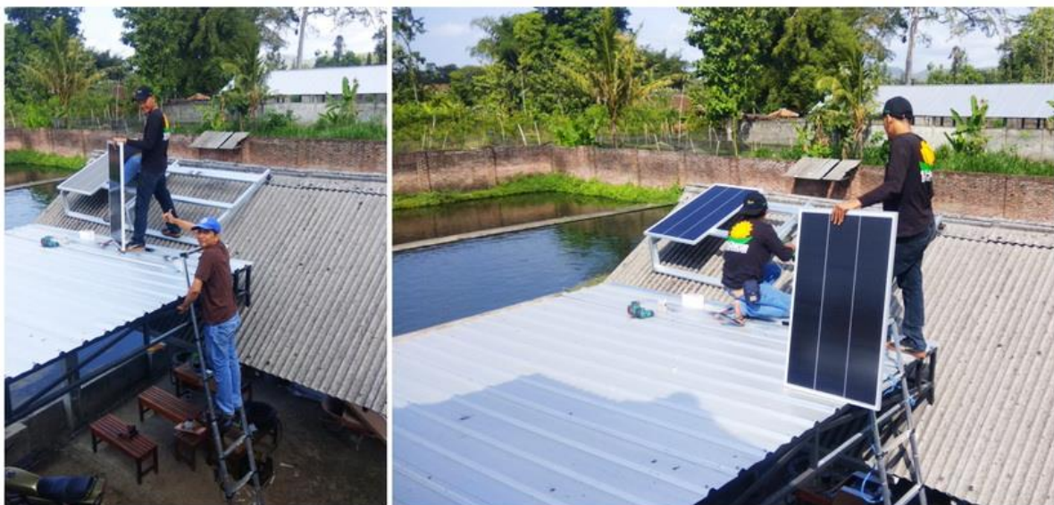
Figure 9. Solar Panel Installation
