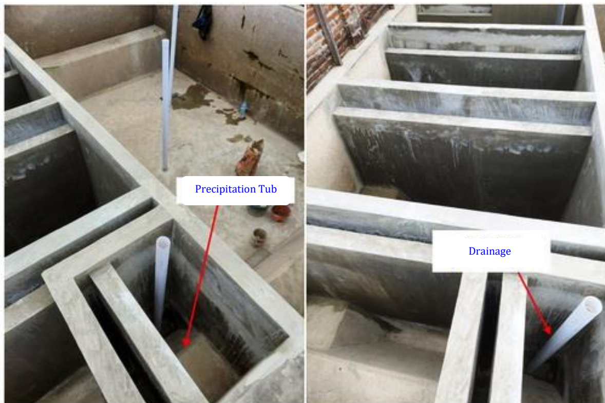
Figure 8. The shape of the tub (chamber) in the Koi. pond filtration system
