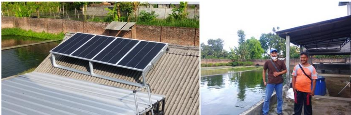
Figure 11. Partner involvement in the installation of 600 Wp Surya solar panels
