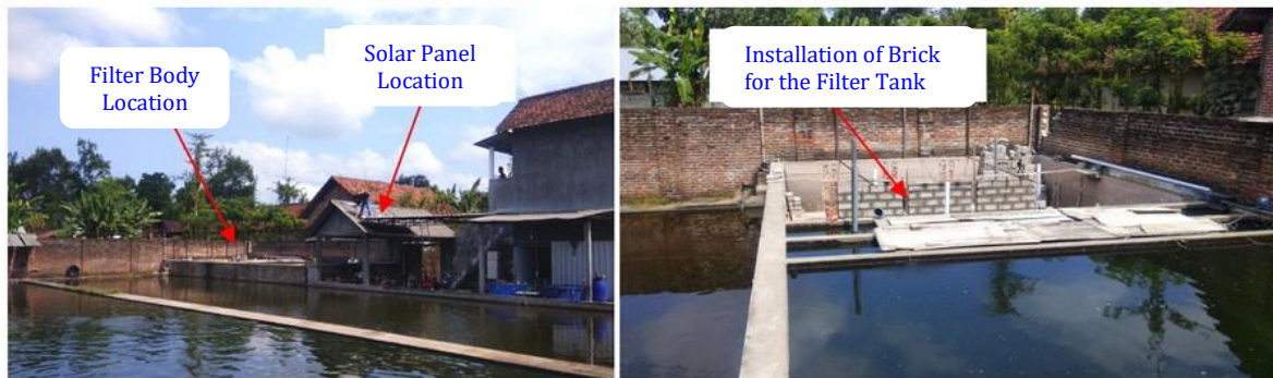
Figure 6. Location of the filter basin and installation of solar panels
