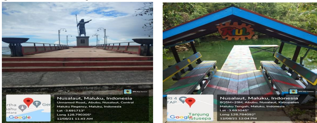
Figure 3. The form of the development of facilities at the Lake Riul object and the MCT Monumen Monument
